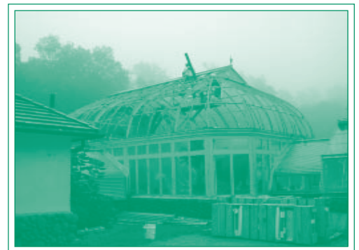
WORKERS REMOVING GLASS AND CLEANING GLAZING BARS.
